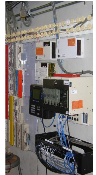
Time Warner Telecom Incoming Service Cabinet and incoming Copper Service Demarc. (Telecom Switchgear Rm)
