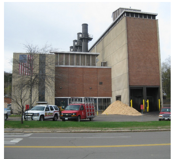
Central Heating Plant
