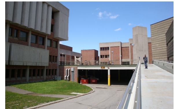
Service dock under Engineering Quad
